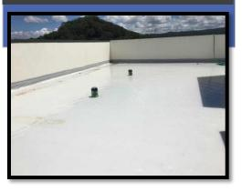
Completion of Sheet Membrane installation Rooftop area of Building 24 & Testing is now complete -
